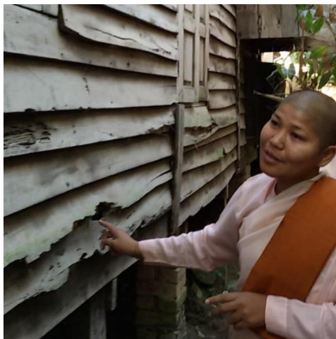
Here in Burma, wood does not last long before being eaten by termites and hollowed out by nesting ants. So old walls need continuous renewal – which they have gotten, thanks to you!
