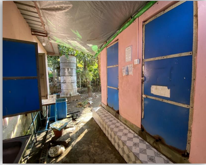
The shower/toilet area
