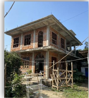
The new building under construction
