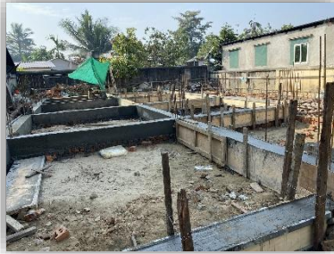
The construction site in January and March 2026
